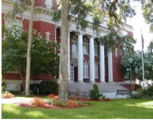
HISTORIC COURTHOUSE HERNANDO COUNTY
