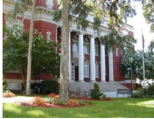
HISTORIC COURTHOUSE HERNANDO COUNTY
