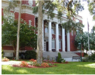
HISTORIC COURTHOUSE HERNANDO COUNTY
