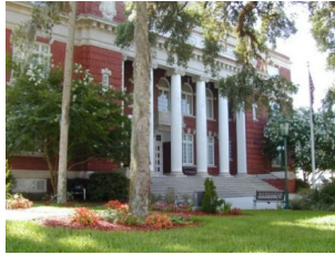
HISTORIC COURTHOUSE HERNANDO COUNTY
