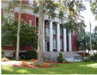
HISTORIC COURTHOUSE HERNANDO COUNTY
