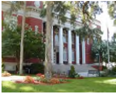
HISTORIC COURTHOUSE HERNANDO COUNTY
