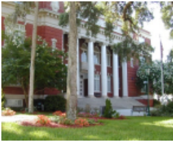
HISTORIC COURTHOUSE HERNANDO COUNTY
