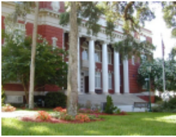
HISTORIC COURTHOUSE HERNANDO COUNTY
