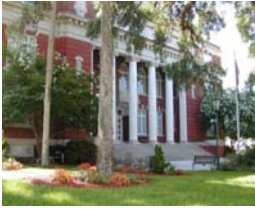
HISTORIC COURTHOUSE HERNANDO COUNTY
